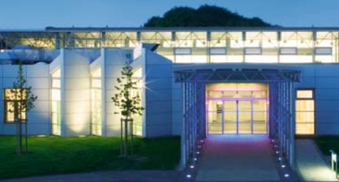
| Customer training centre, Lüdenscheid
