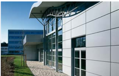
Customer training centre, Lüdenscheid
